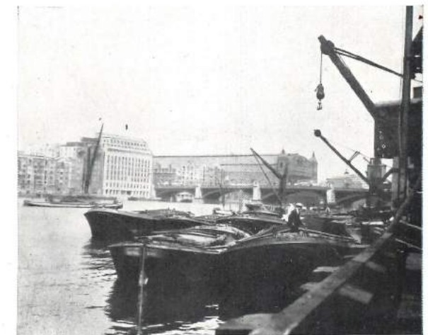
View looking from Bankside.
