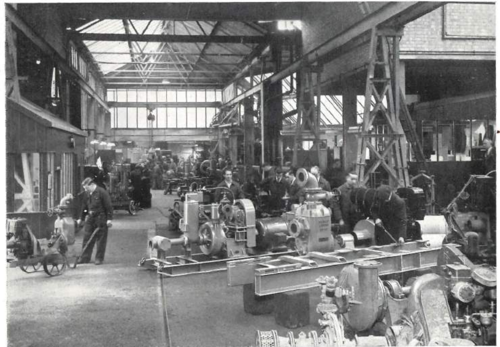
General view of Assembly Shop, Southwark Street Works.
