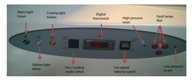
TLZ 11 Thermostat Press button De P once and release. Set point value and set point will be displayed alternately. Press Key to change the value of the set point. Once the desired value is displayed press P again to memorise the set point.
