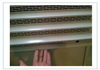
To access filter, lift the return air grille and remove panel. Clean filter in warm soapy water, shake dry and replace ensuring filter is positioned correctly.
