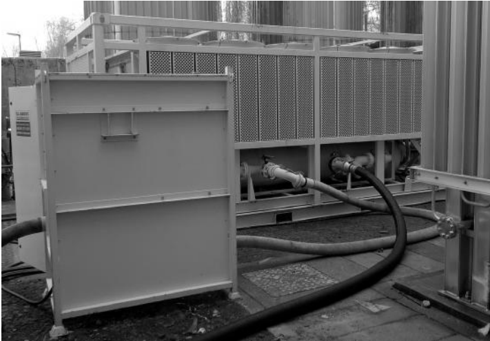
Fig 2 : External pump to pump into the system and then the system return pipework to connect onto the return connection on the chiller. In-line water strainer on the return connection.
