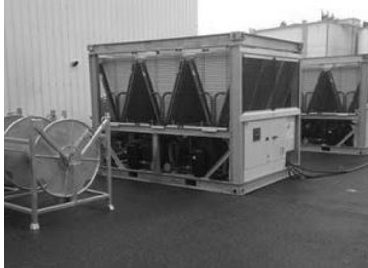
Fig 3: When it comes to filling the system with water you can back fill the chiller and hoses from the customers system or connect an external hose to the chiller via the fill point on the internal pump.
