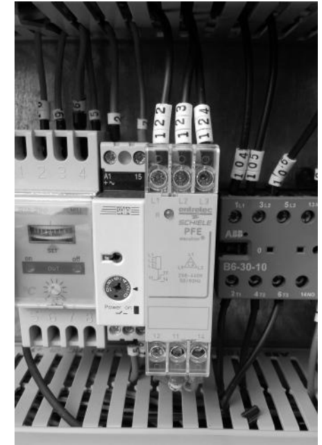
Fig 4: If phase rotation is incorrect then the controller will not light up and the unit will not work
