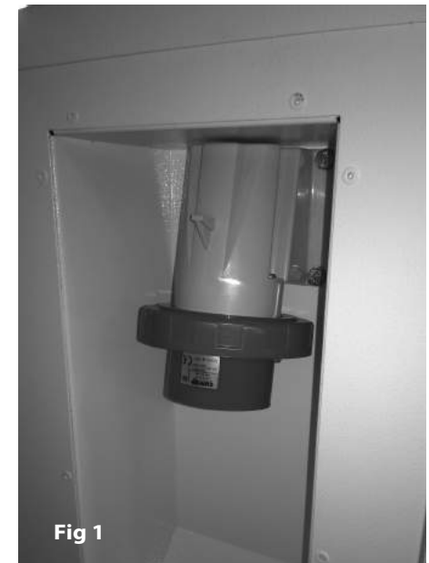
Fig 1 5 pin 32amp 415 volt Appliance inlet plug found on the HPAC 30
