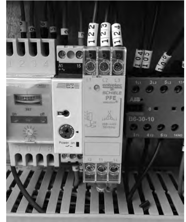
Fig 4: If phase rotation is incorrect then the controller will not light up and the unit will not work
