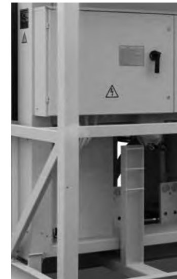
Fig 1: Cable entry tray is positioned below main isolator switch. 4 x 95mm cables required for hard wired connection.
