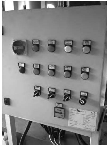
Fig 5: Example of the switch gear control panel
