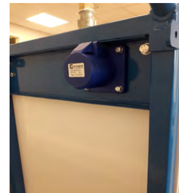
Fig 1 : Phase rotation does NOT need to be checked with this 415v appliance
