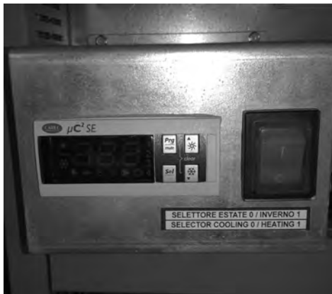
Fig 5: Carel 4 button controller Red switch position 0 Cooling selection Red switch position 1 Heating selection
