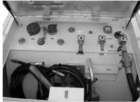
Fig 4: Pressure and temperature gauge for boiler monitoring. manual reset pressure switches
