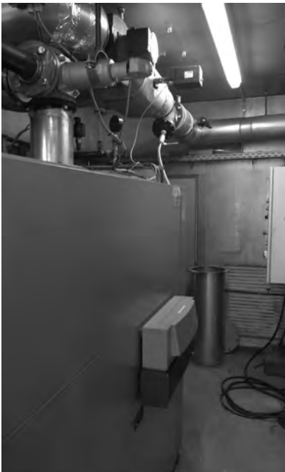
Fig 3: The boiler control panel for boiler temperature control The 1250kW boiler doesn't have a plate heat exchanger so no primary or secondary sides
