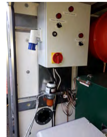
Fig 1 : 240 volt Appliance inlet plug Cable entry is through the black round port hole below the control panel
