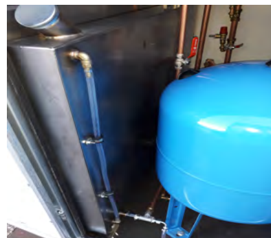
Fig 6: Internal fuel switcher valve to switch from internal to external fuel tank
