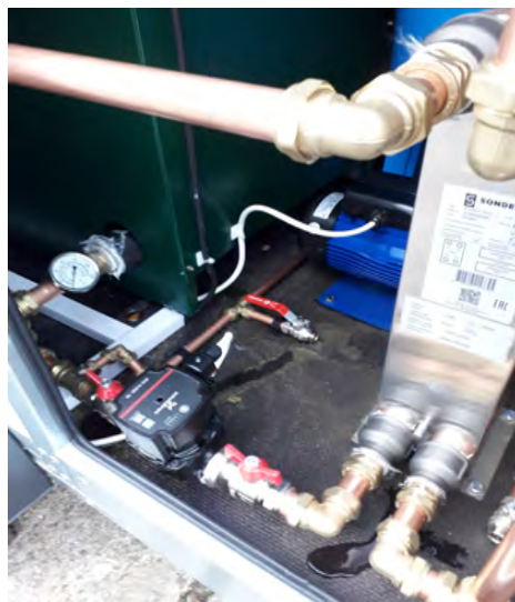
Fig 3: The 100kW Rapid Response Boiler has a heating only plate heat exchanger. The primary side of the heat exchanger will need to be filled with water to 1.5 bar
