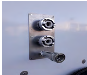
Fig 5 : 2 x 1" storz connections for flow and return heating connections Fuel connection for external tank
