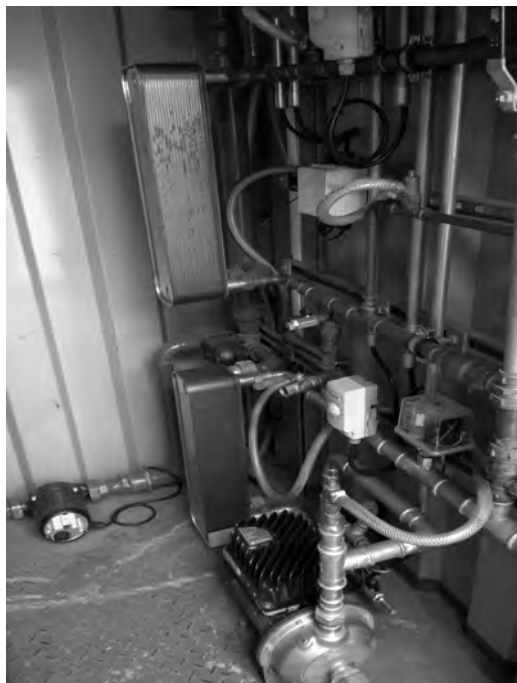
Fig 3: The 100kW Packaged Boiler has heating and DHW plate heat exchanger. the primary side of these heat exchangers will need to be filled with water to 1.5 bar
