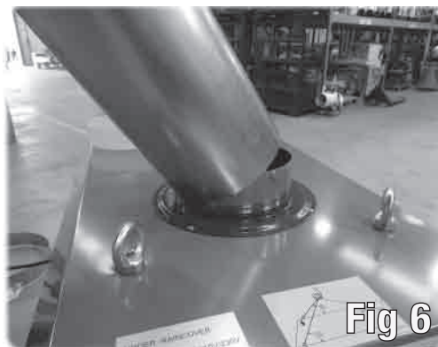
Fig 6 : Remove protective cover and fit flue gas exhaust pipe (1 metre) onto the outlet flue gas supply spigot
